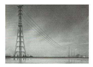
Where power lines need to cross water, a different design of pylon is needed. They have huge height extension to give them the ability to span the river with the wires.
