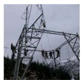
It's necessary for a team of men to climb the structure in order to secure each part in place. Then the wires are added and tensioned.
