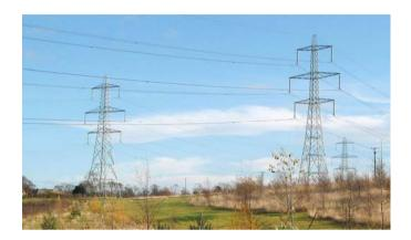
The most commonly seen pylons in the UK are the L2, L6 and L12 series. We have already covered the L2, identified easily by all the arms being the same width.
