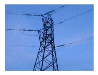
Where power lines have to turn a corner, you need a deviation pylon!
