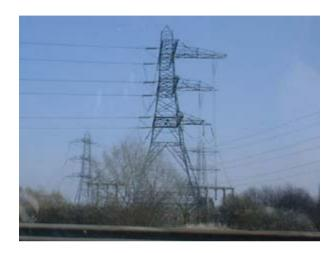
Terminal pylons are used where power lines end. Perhaps they terminate at a substation, or continue their journey underground.
