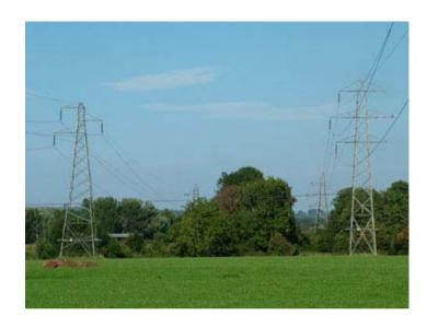
Before 1928, we did not have any standard pylon designs in the UK. A competition was run by the Central Electricity Board. The winning design was chosen by the architect Sir Reginald Blomfeld and became the series PL1 and PL1b.
