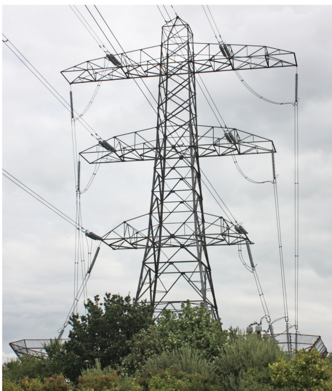
L2 DT terminal tower, Chingford, North East London
